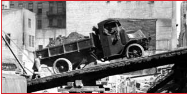
Hard At Work On New York Subway System
